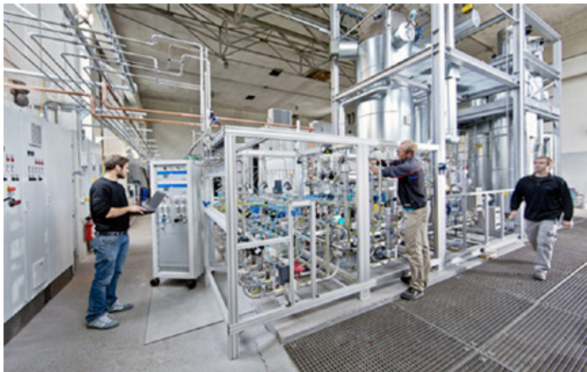
Pilotanlage Power-to-gas in Stuttgart (m.technologyreview.com)
